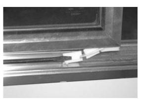
• Step 4: Pull the screwdriver handle away from the panel to disengage the guide from the track allowing you to further adjust the roller brackets.
