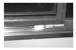
• Step 2: Place the narrow side of a flat head screwdriver into the guide's groove so that at least half of the screwdriver's flat side is flush against the guide.
