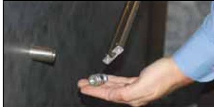
Insert Aluminum Slide Fittings into the Railing
